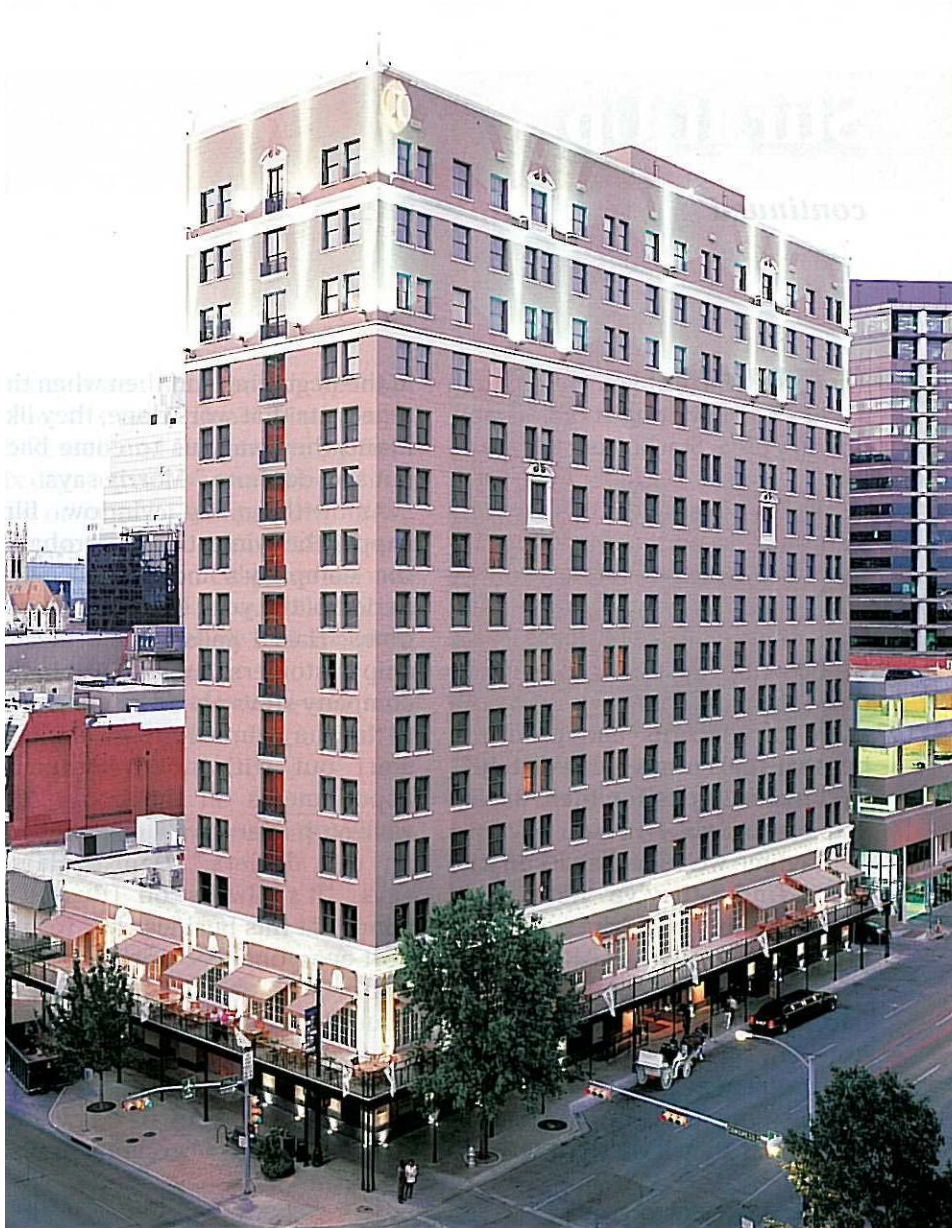
Sun Tint applied Solar Gard Stainless Steel 50 to the Stephen F. Austin Hotel (shown here) in Austin, Texas.
