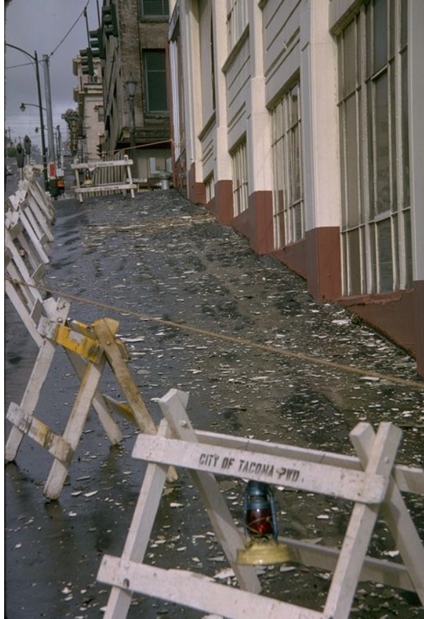
Figure 1.2 Damage to window systems observed during the Puget Sound, Washington, 1965 earthquake. (Courtesy of the National Information Service for Earthquake Engineering, EERC, University of California, Berkeley)
