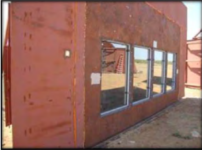
Figure C.1: Chamber 1 Pre-Blast Condition
