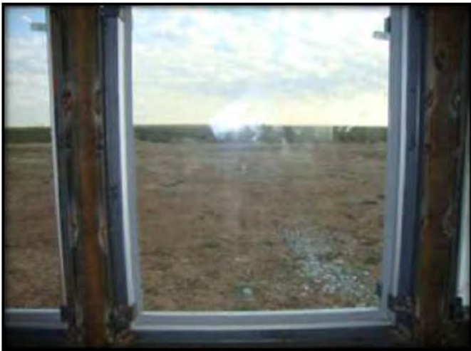
Figure C.27: Specimen 15 Internal Post-Blast Condition
