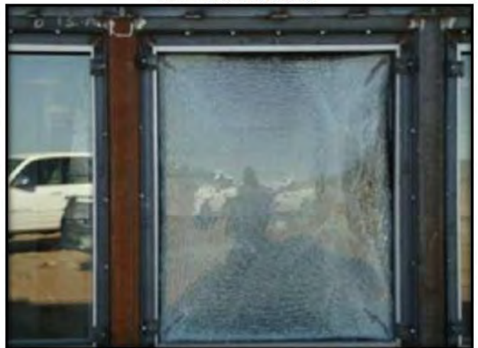
Figure C.22: Specimen 14 External Post-Blast Condition
