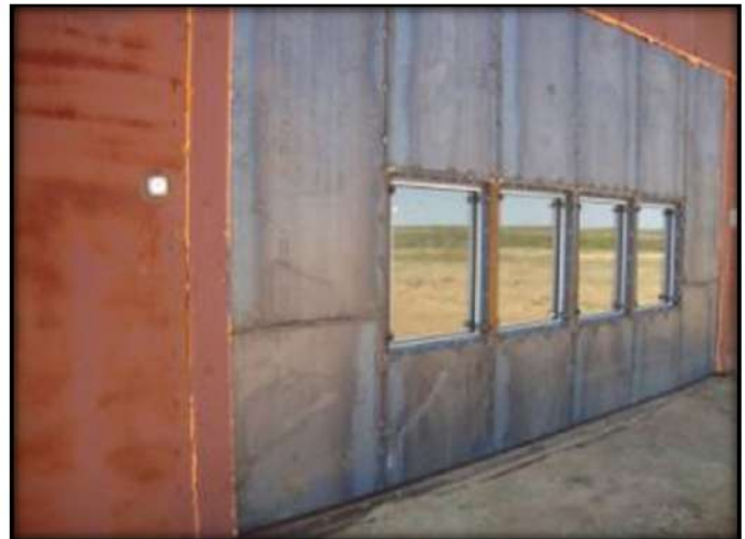
Figure C.16: Chamber 4 Pre-Blast Condition
