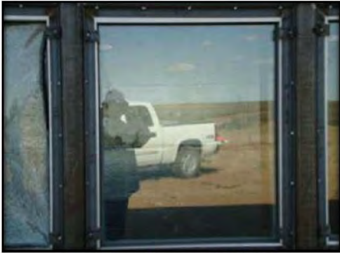
Figure C.23: Specimen 15 External Post-Blast Condition
